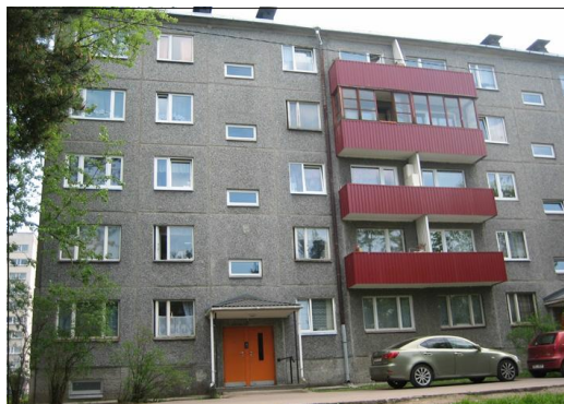
Figure 7: Major renovation in one case study apartment building in Tallinn; before (left) and after (right).
