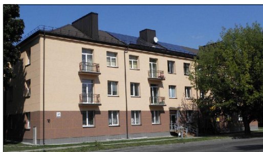
Figure 8: Multi-apartment building renovated using the JESSICA financial scheme.
