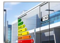
Figure 8: Example of EPC displayed in an office building.
