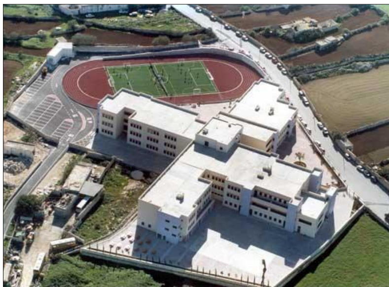
Figure 6: Energy efficient secondary school building at St Benedict's College, Kirkop, Malta.
